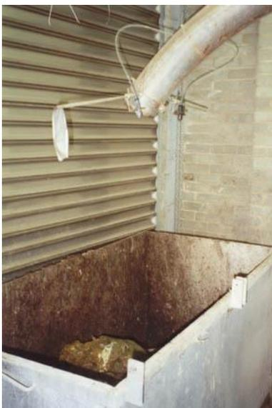
Untreated sewer from initial stage of treatment. triple<sup>7</sup> Odour Control is misted over bin by nozzles attached to outlet pipe.
